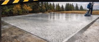
CONCRETE RESTORATION & EPOXY COATING
